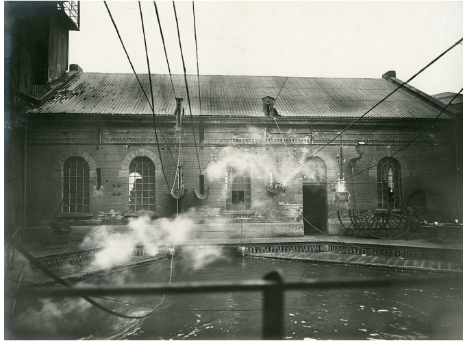
A wire rope power transmission leaves a water power plant, heading for a paper factory in Heilbronn, Germany. The line, 90 m long, was constructed in 1888. Photo credit .
