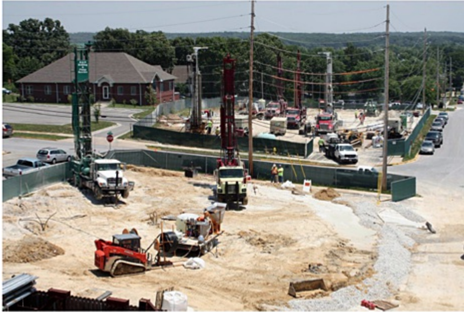
Figure 4. The use of multiple rigs to speed operations (how many?) (MST)
