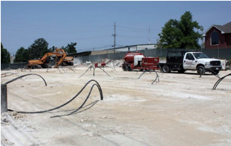
Figure 5. After pipe installation (MST)
