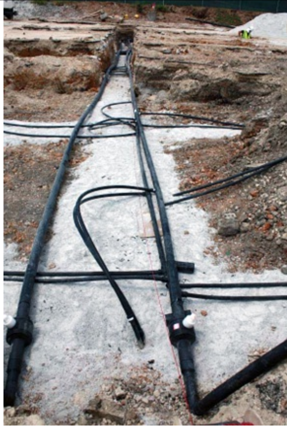
Figure 6. The connections between the wells and the distribution network. (MST)
