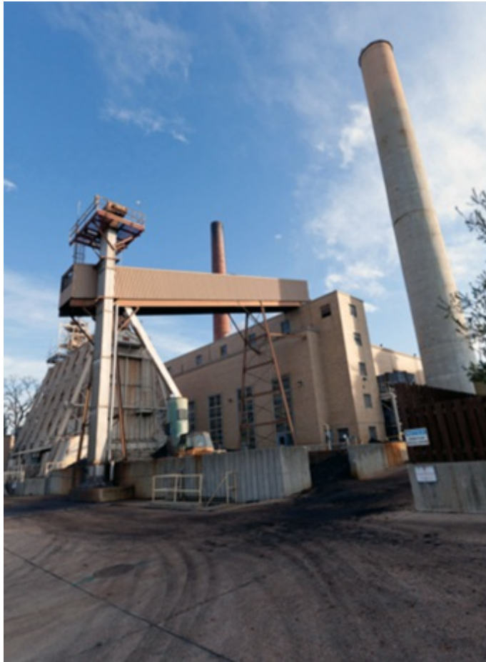
Figure 2. Old Campus Power Plant - the question of what to do with the stacks is unresolved.
