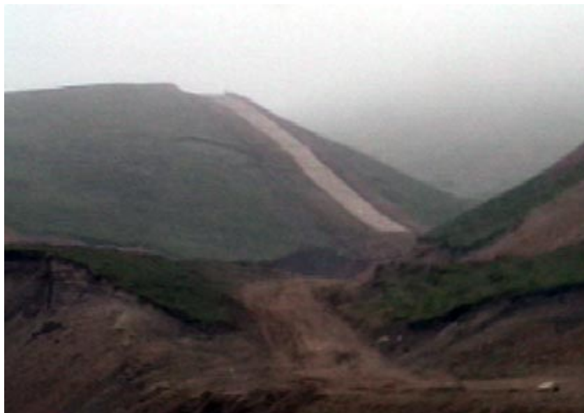
Figure 3. New gas pipeline being laid in China in 2009.
