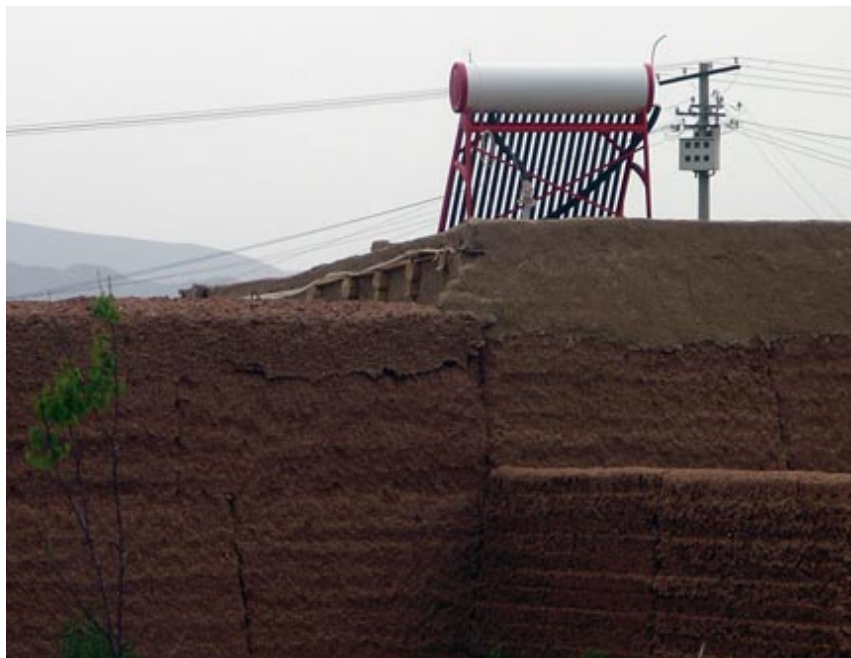
Figure 7. Solar water heater (cost around $1,000 installed)
