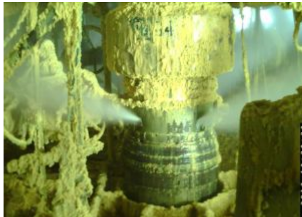
Figure 7: Leaking Elgin wellhead
