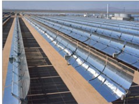
Parabolic trough collectors.
