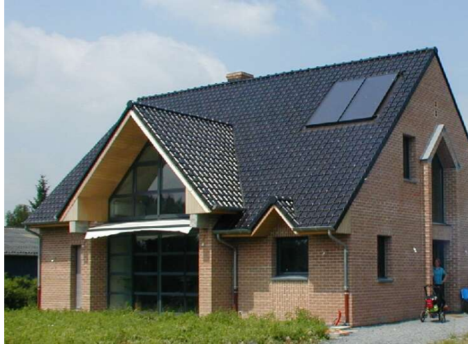
Two panels on roof provide hot water.
