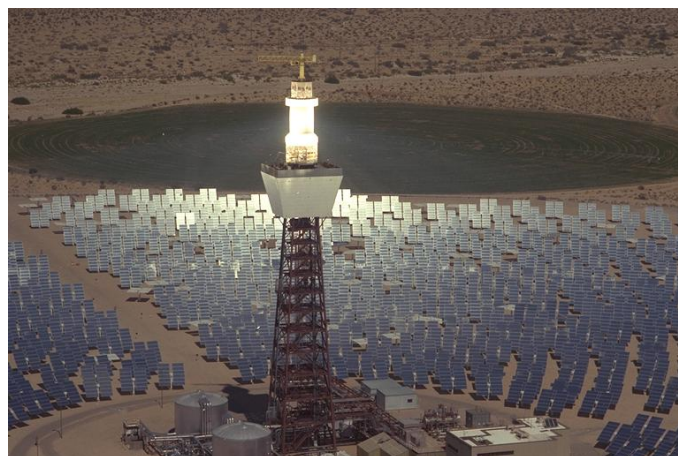
Solar "power tower" outside Barstow, CA.
