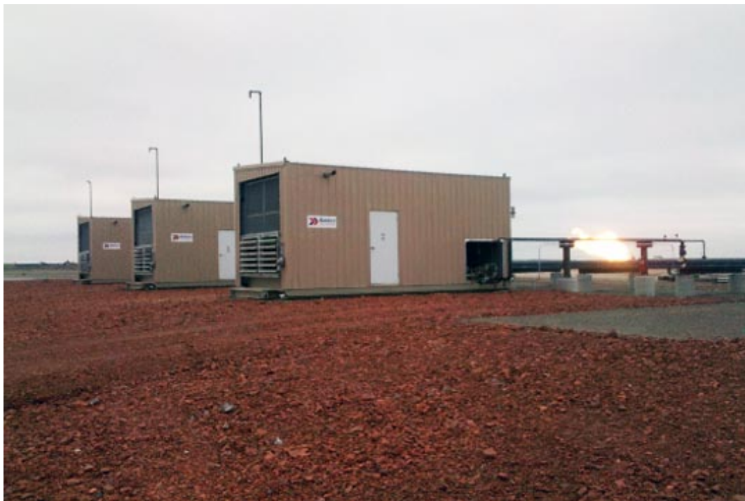
Skid mounted compressors at a well, separating and compressing the gas. ( Bakken Express )
