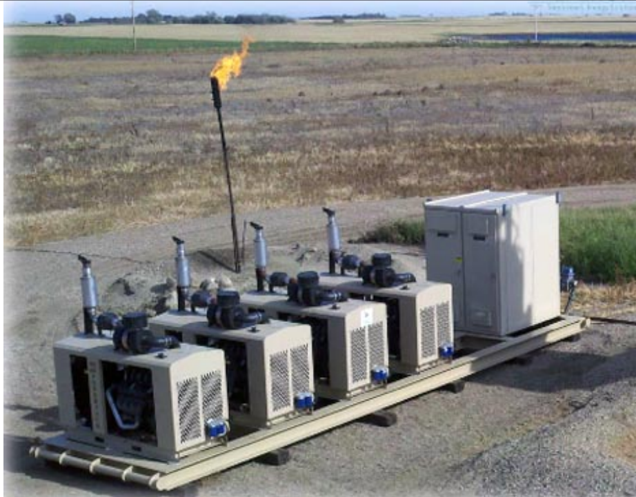
Generators at a well site, using the natural gas to generate electricity ( Blaise Energy ).
