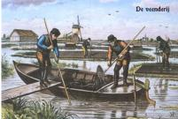
However, now that it was possible to cut peat far below the water level, the complete peat bogs could be mined. There is evidence that the "baggerbeugel" was already in use in Flanders two centuries earlier, and that the knowledge of the technique was transferred to the North.
