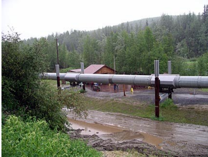
Alaskan pipeline just North of Fairbanks. Note the radiators on the support legs. These disperse the heat from the pipe (and the oil) which keep the permafrost, in which the support legs sit, from melting. The 48-inch line was sized to carry 2.1 mbd of oil. Today it only carries around 660,000 bd .
