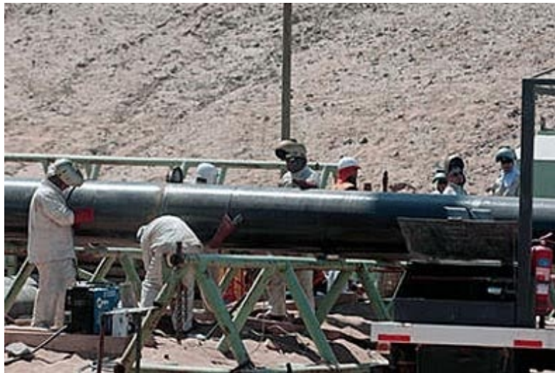
Preparing the casing for the shaft
