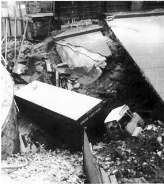
(Photos courtesy of Mott McDonald)
