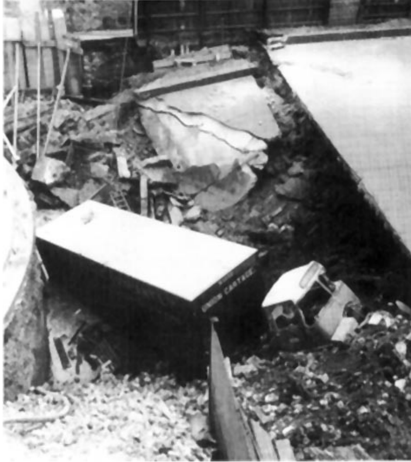
(Photos courtesy of Mott McDonald)
