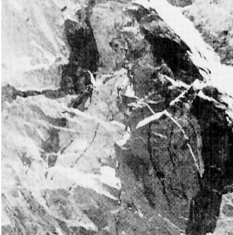
Rock after grouting (white lines)
