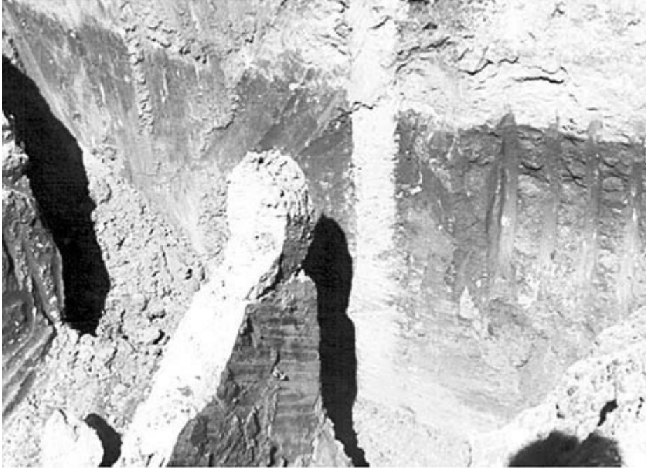
Grout wall exposed to show the 12-inch thickness and integrity.
