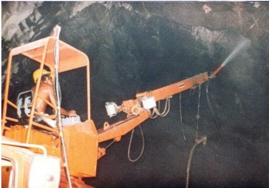
Applying shotcrete with the operator well back from the face ( Evert Hoek )
