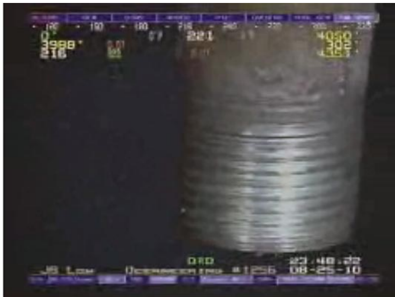
Close-up of the lower end of the pipe
