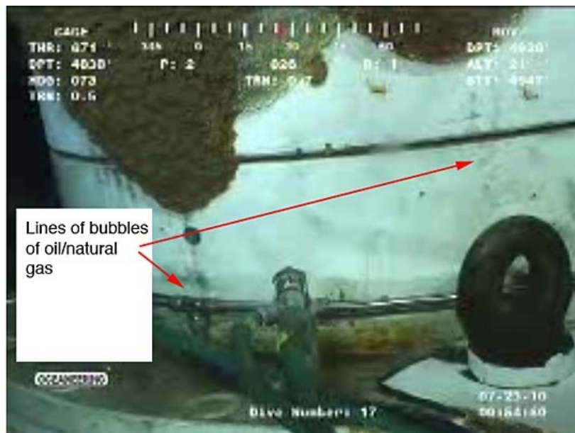
Leaks on the fittings around the wellhead
