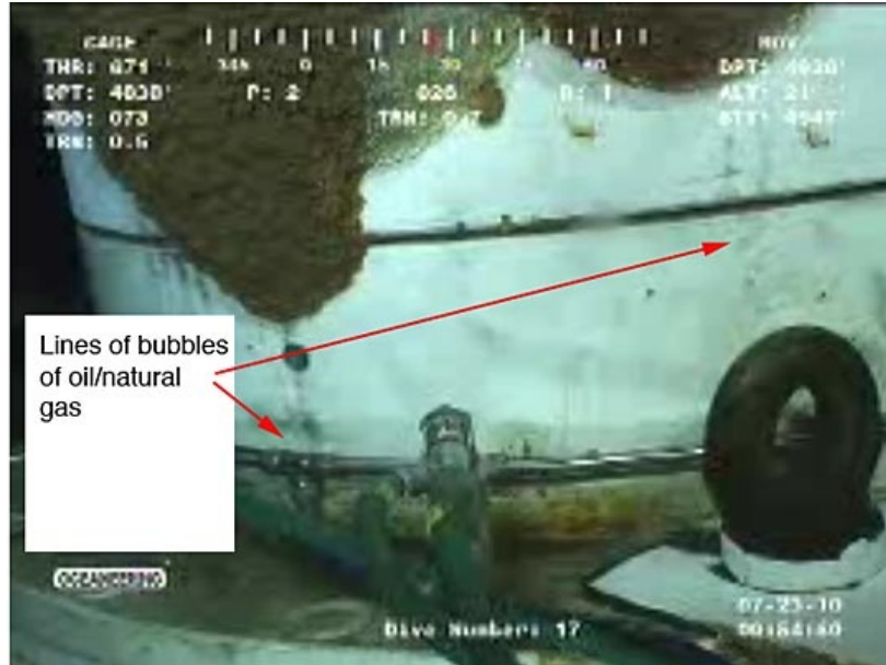
Leaks on the fittings around the wellhead
