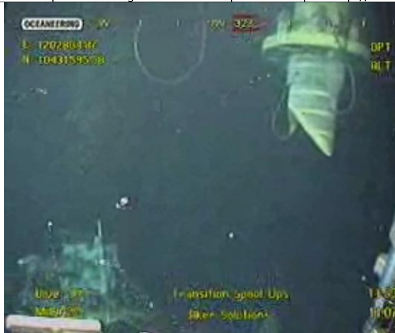
Transition spool approaches the flowing well
