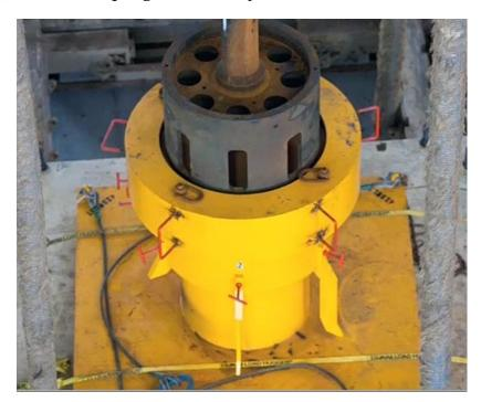
This will expose the two segments of drill pipe that are sticking out of the BOP, and so these will then be strapped together, so that they will fit within the transition spool. A guide shoe and positioning pins will be used to help lower this in place, and then the ROVs will bolt the 12 ft flange transition spool (the yellow segment) to the top of the old BOP.
