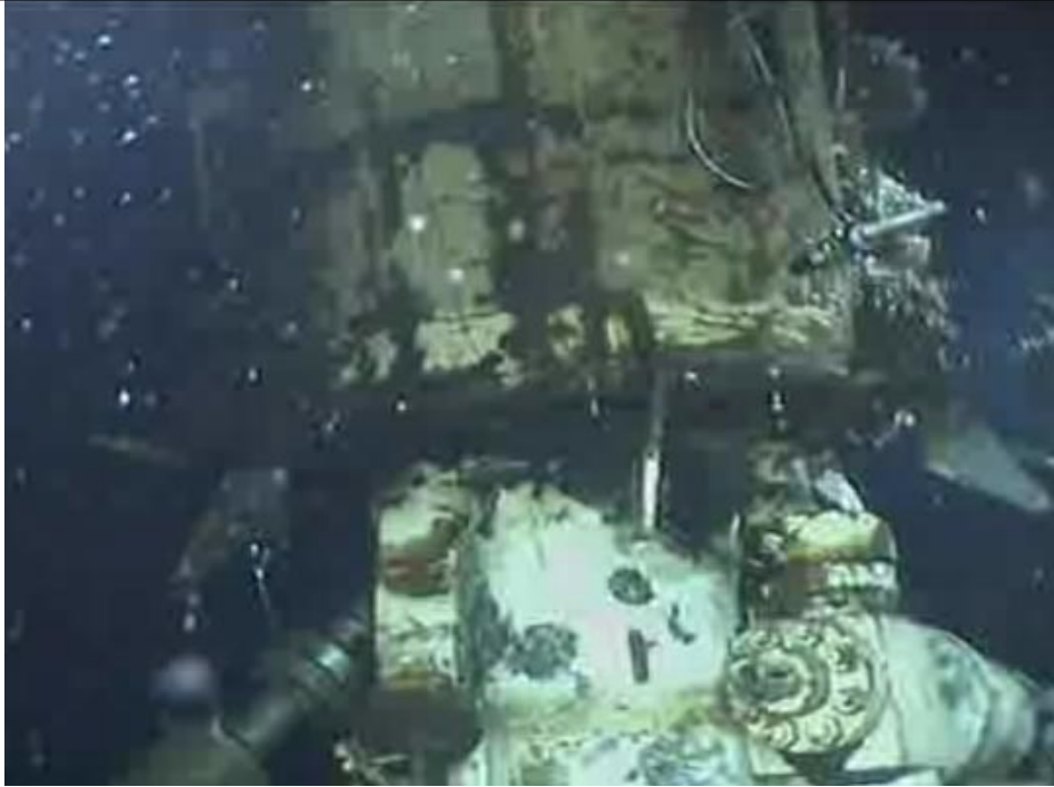
View of the cap 9:50 pm June 24, showing no leak on the Enterprise ROV side of the cap.
