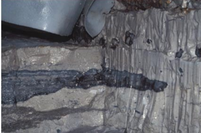
Dolomite and chert cut with an ASJ in the walls of the Omnimax Theater under the Arch in St Louis. (Its all hidden behind the concrete wall now).
