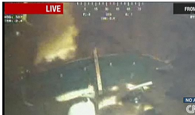
Leakage around the seal between LMRP 7 (yellow), the seal (greenish black) and the LRA. (white)
