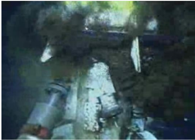
Leaks under the LMRP at 10:30 pm
