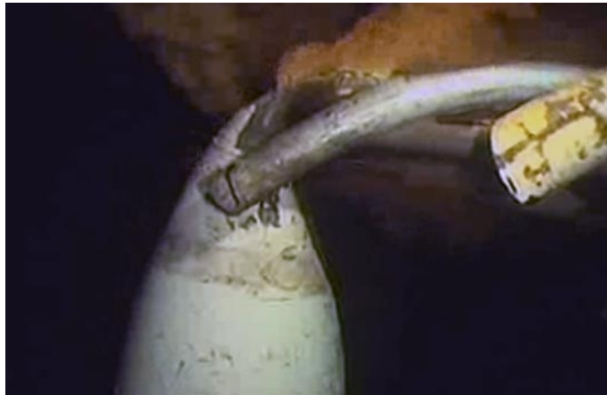
The wire saw was then located ready to make the cut.
