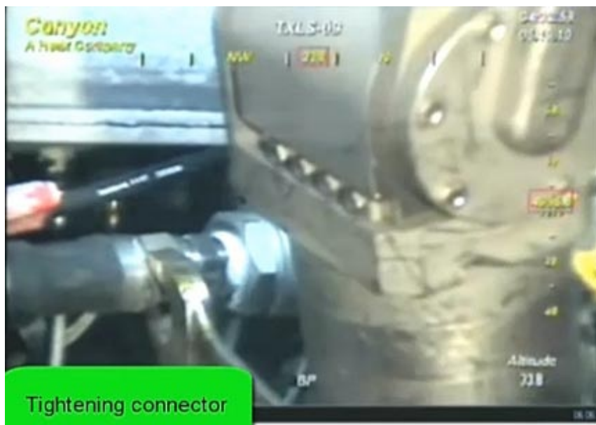
ROV image showing the control pod fitting being tightened
