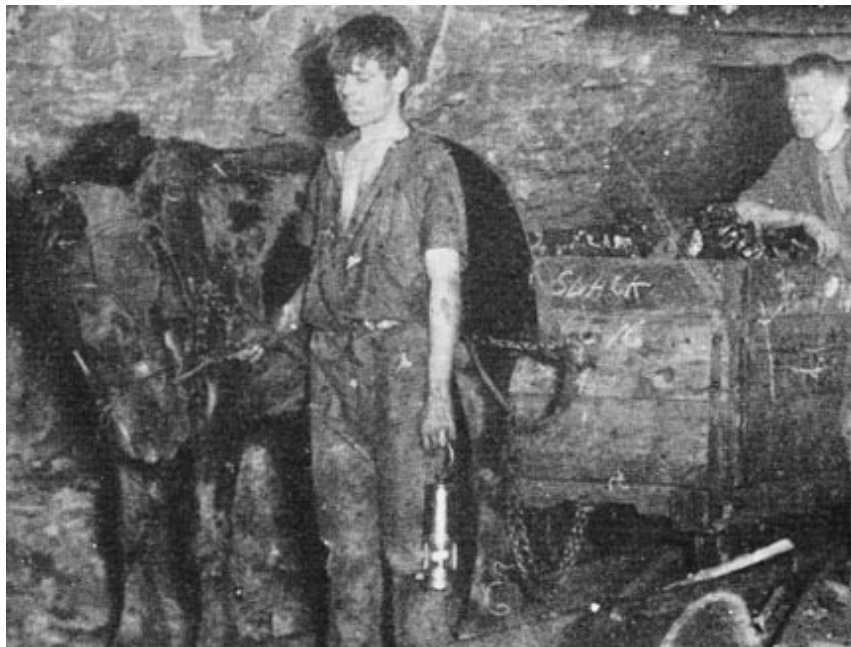
Pony hauling a tub full of rock (slack - coal contaminated with rock or other dirt) (From “The
