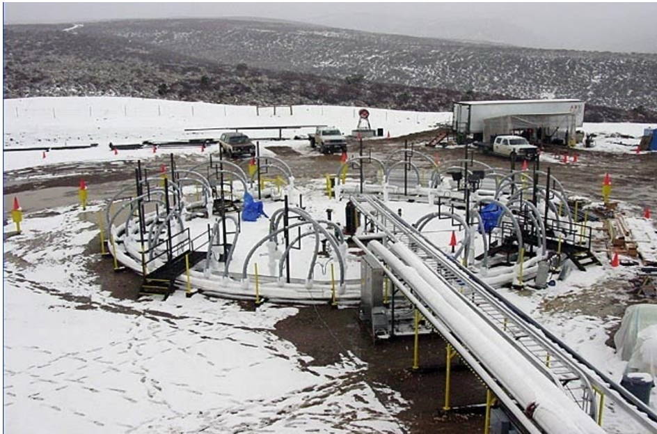
Shell freezing test
