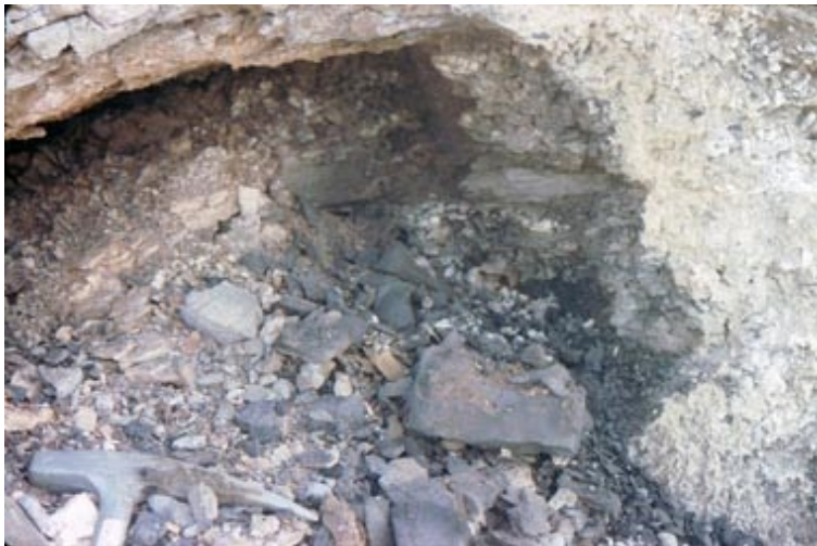
Collapsed cavity where high-temperature overlying shale fragmented and “blew out” after being hit by a water stream. (site in Montana)
