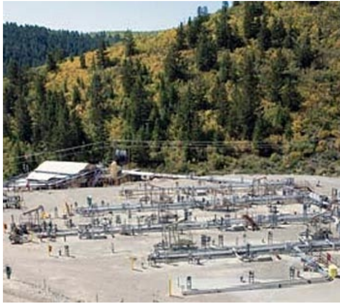
Array of heaters at a Shell test site
