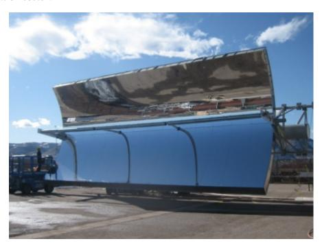
Parabolic troughs focus sunlight on liquid-filled receivers suspended over the mirrors to create steam that drives an electricity-generating turbine. Parabolic trough technology has been in modern use in solar power plants since the early 1980s, but Alcoa executives said they saw an opportunity to refine the technology and get a foothold in the rapidly expanding renewable energy market.
