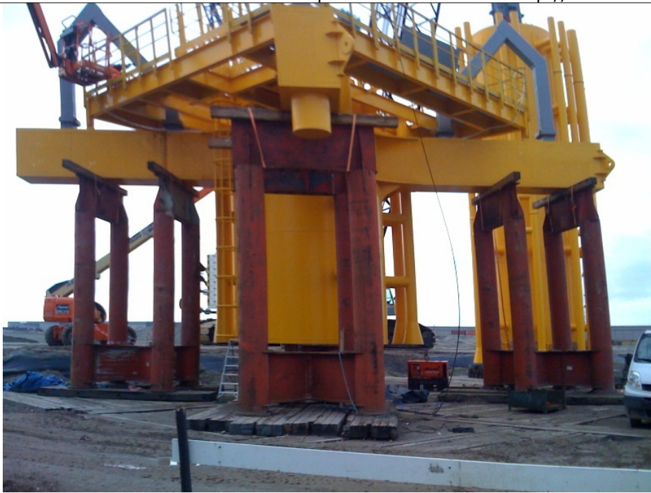
the transition piece for the offshore high voltage transformer station
