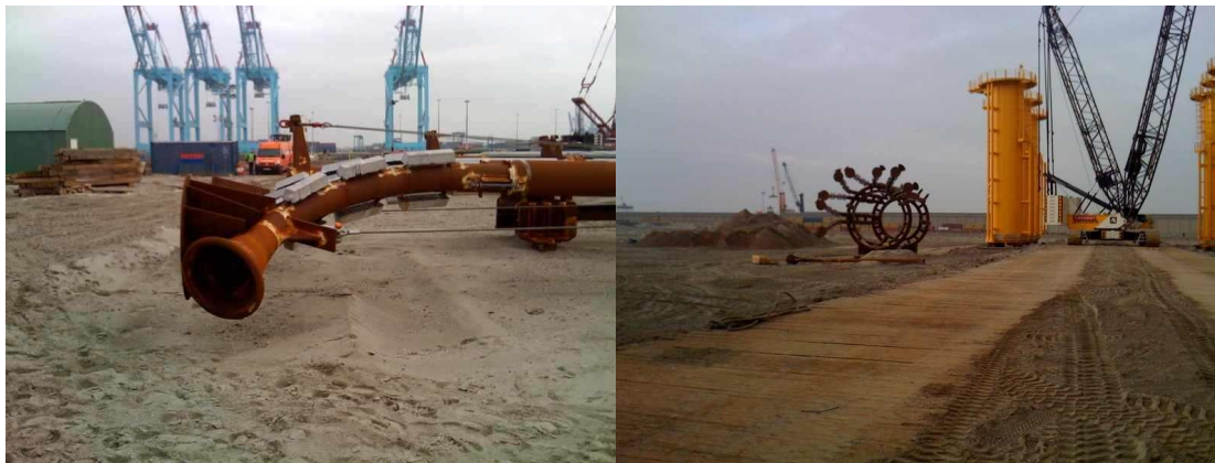
On the left, you can see the bottom part of the j-tube, while the right picture has the more complex set of j-tubes for the transformer station, which has several cables going to several "strings" of turbines. Note the anti-corrosion protection on the j-tubes.
