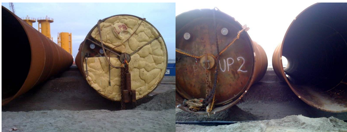
the two plugs used to float a foundation,
