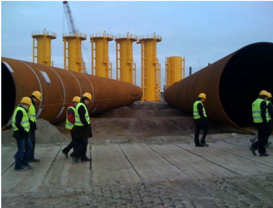
two foundations on the ground with several transition pieces in the background
