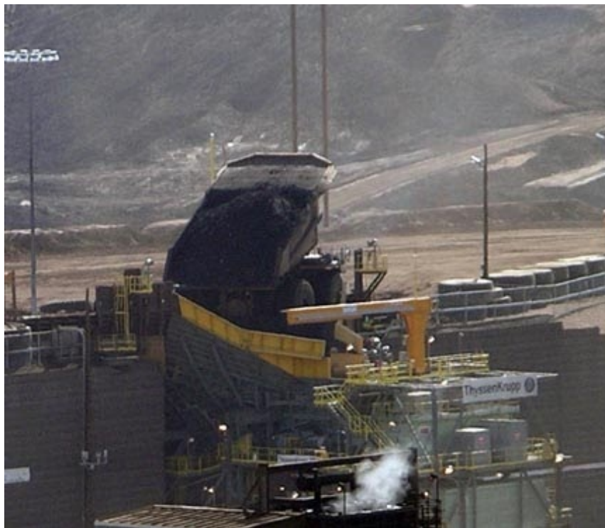
Tipping into the breaker
