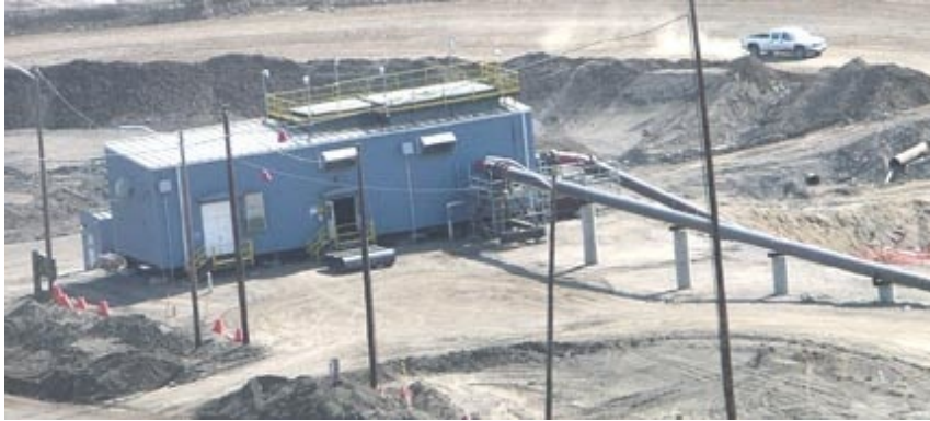
Pump station and delivery pipeline
