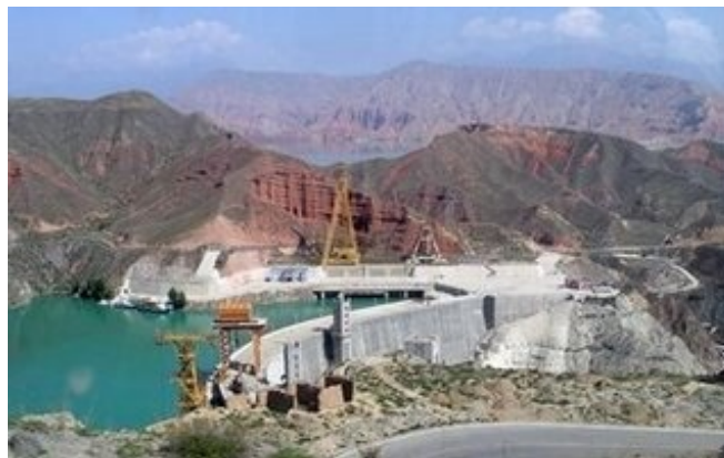
The Liujia Gorge dam and lake
