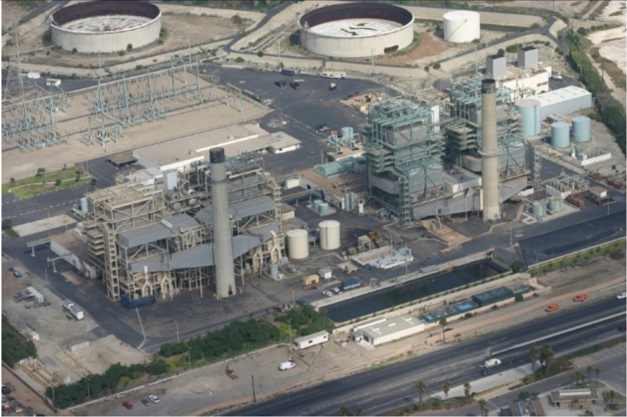
Figure 3: AES 450 MW natural gas power plant, Huntington Beach, CA
