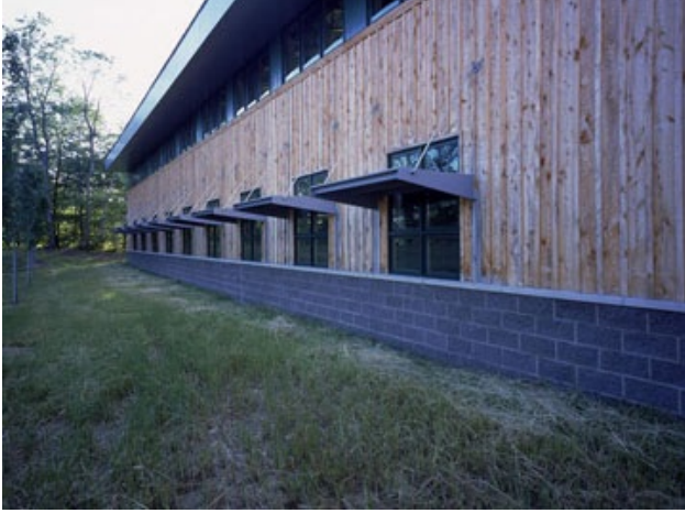
Figure 25 - Overhangs doubling as light shelves
