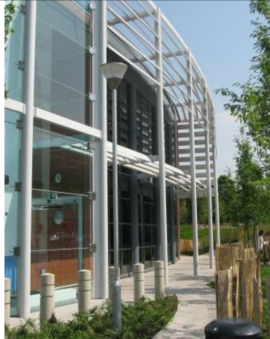
Figure 22 - Multi-story louvered overhangs
