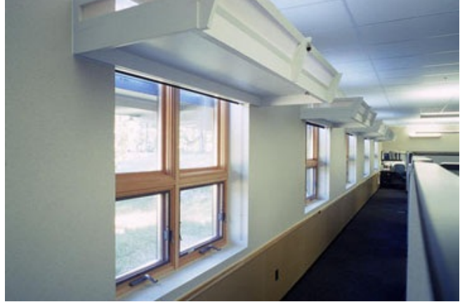
Figure 26 - Light distribution from light shelves
