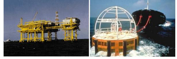
The Marine Terminal (yellow structure in the above image) coordinates vessel traffic in the vicinity of the LOOP, maintaining safe distances between tankers. For oil offloading, tankers are tethered to one of the moorings and flexible hoses bring oil from the tankers and pass it into one of several sea-floor pipelines spanning the 20 mile distance to the Fourchon Booster Station located onshore.
