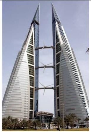
Taking architecture, and wind power, to new heights, developers of the Bahrain World Trade Center in Manama, Bahrain, flipped the switch to start three huge turbines set between two towers — a first glimpse of technology that they hope will power up to 15 percent of the center.
