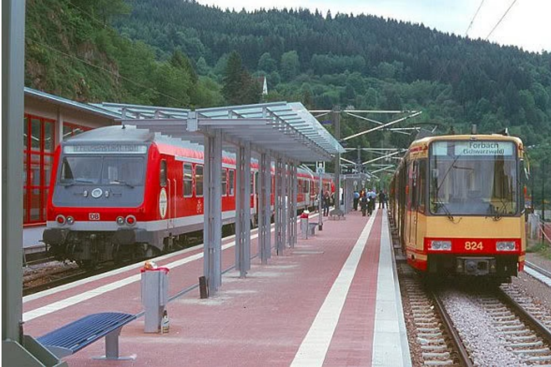
Meeting in the freshly renovated Forbach-Gausbach station on May 18th, 2002: left a push-pull stopping train in limited-stops service, right dual-system tram No. 824 of Karlsruhe's Stadtbahn .
