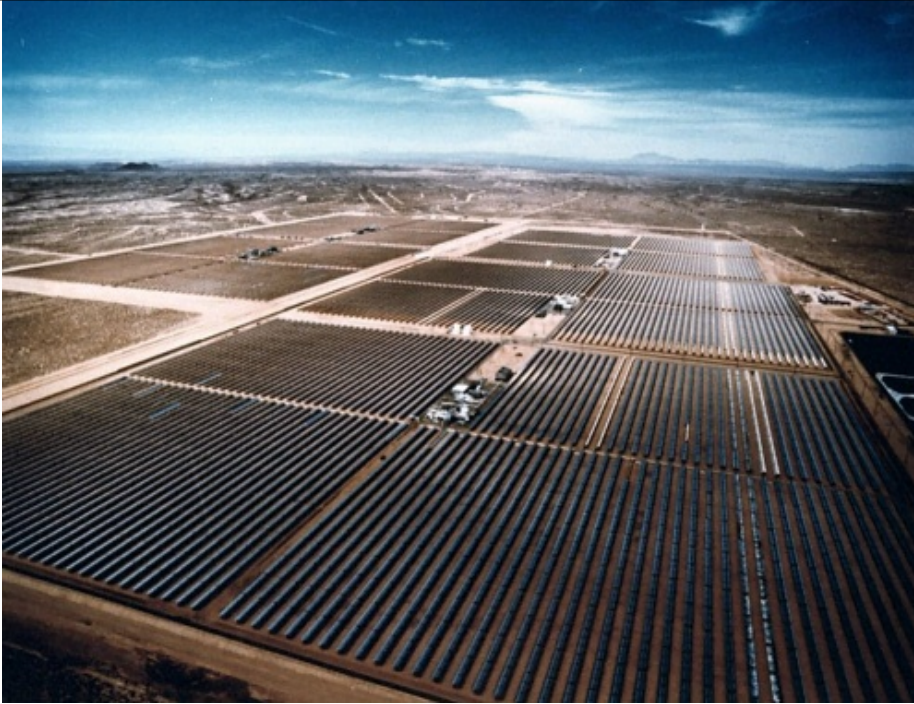
150 MW of parabolic trough CSP plant at Kramer Junction, California.
