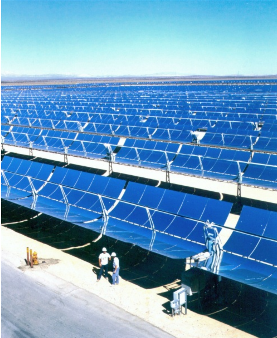
Parabolic trough mirrors with maintenance workers at Kramer Junction, California.
