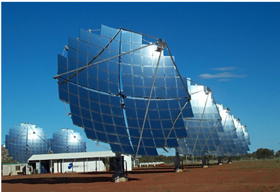
Dish/engine systems from Solar Systems at Umuwa, South Australia
