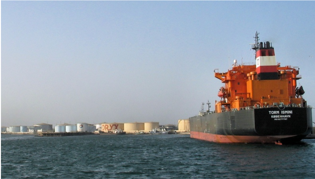
Oil storage tanks at Dakar.
