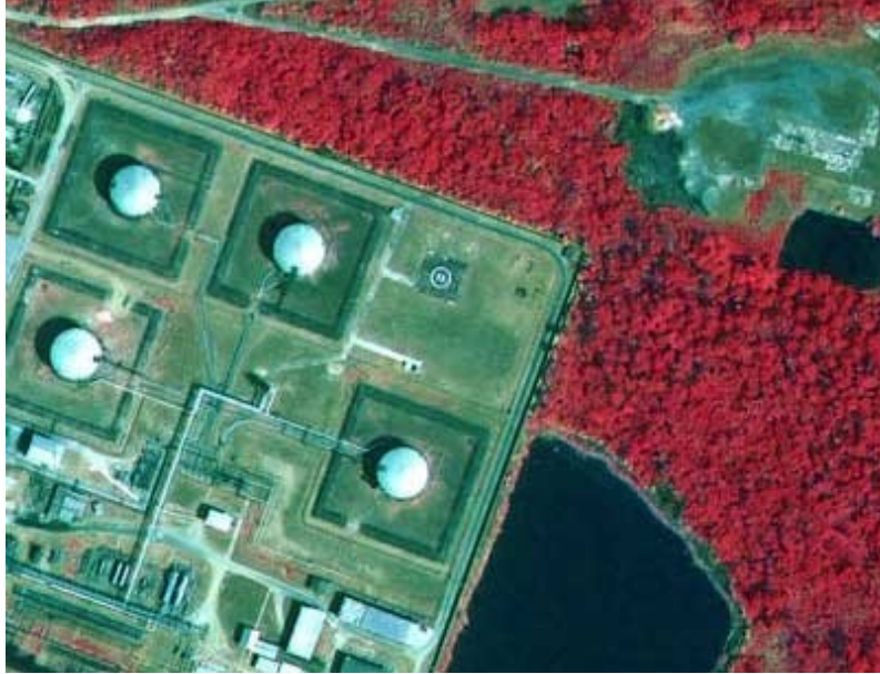
Figure 7: Hyperspectral Satellite Image of Oil Installation in Nigeria—Note dense jungle in close proximity to facility perimeter, a result of economics-driven design.
