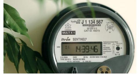
Being adaptable remotely allows the utility to alter the hours designating peak, intermediate and off-peak price bands in order to accommodate a different usage pattern on weekends and also seasonal variations in peak demand. As meters can also be read remotely, there will no longer be a need for a utility employee to visit in order to read the meter, and there will be no more estimated bills.
