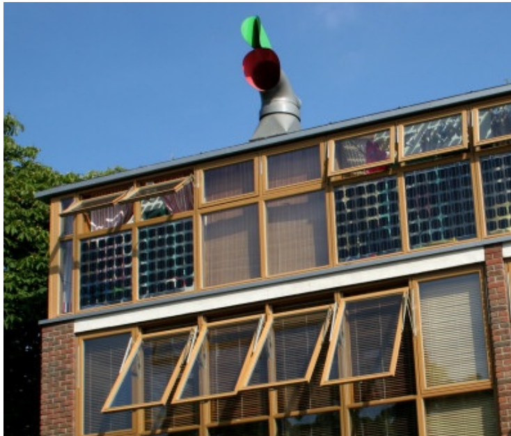
This is a photo I took last year at BedZed showing the photovoltaics in the upper windows with the dual purpose of generating electricity and providing shade. Click to enlarge .
